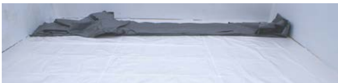
Figure 33 – Despliegue del liner
