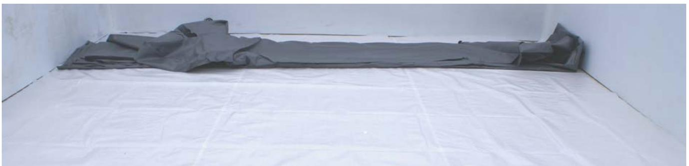
Figura 33 – Unfolding the liner
