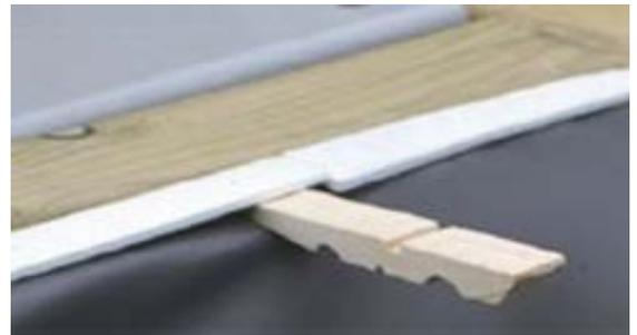
Figura 32 – Blocking the liner in position using half clothes pegs
