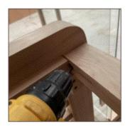
7. Position the vertical supports using the pre-installed cleats
